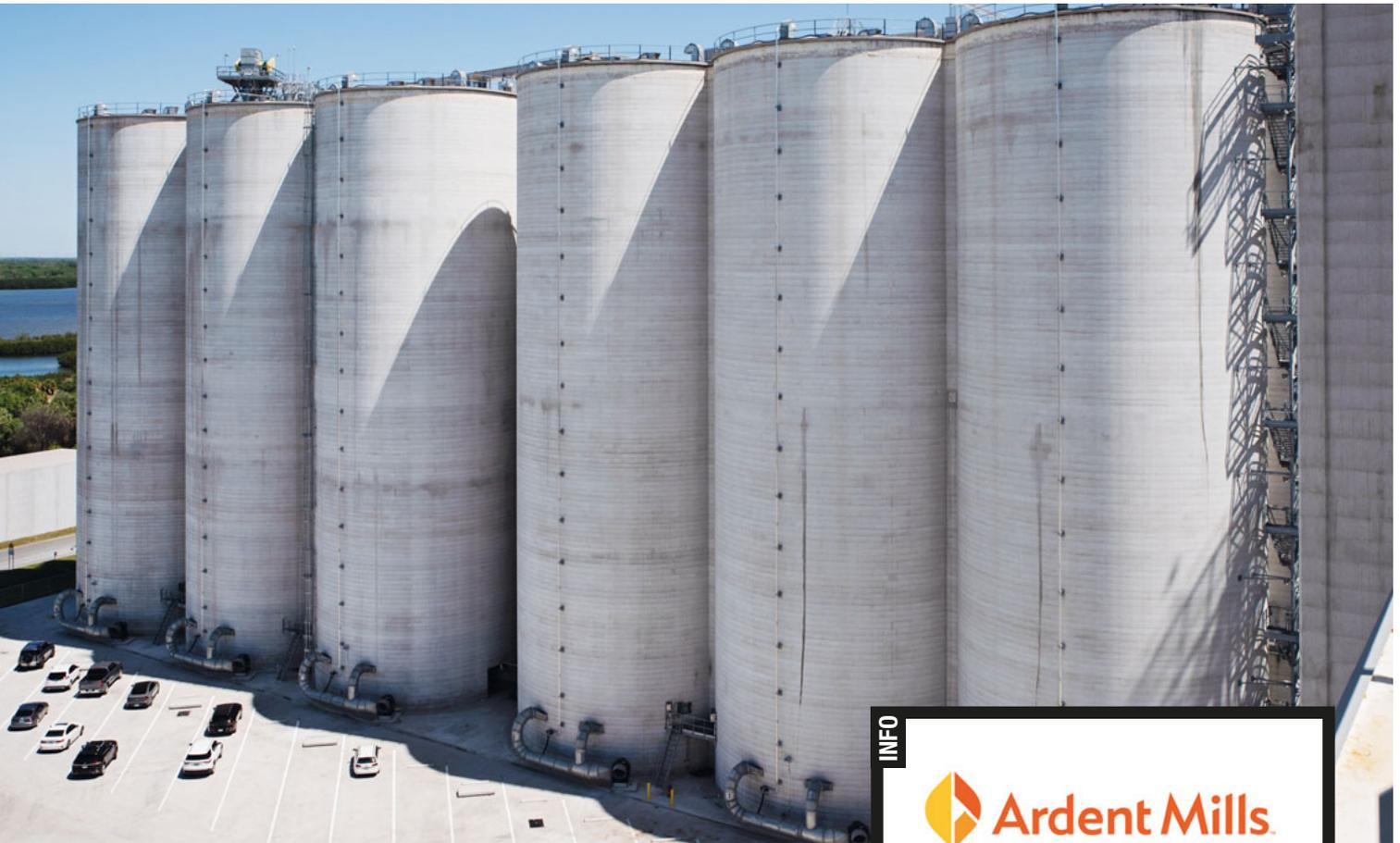
The 160-foot (around 50 meters) silos have a total storage capacity of 111,000 tonnes.
