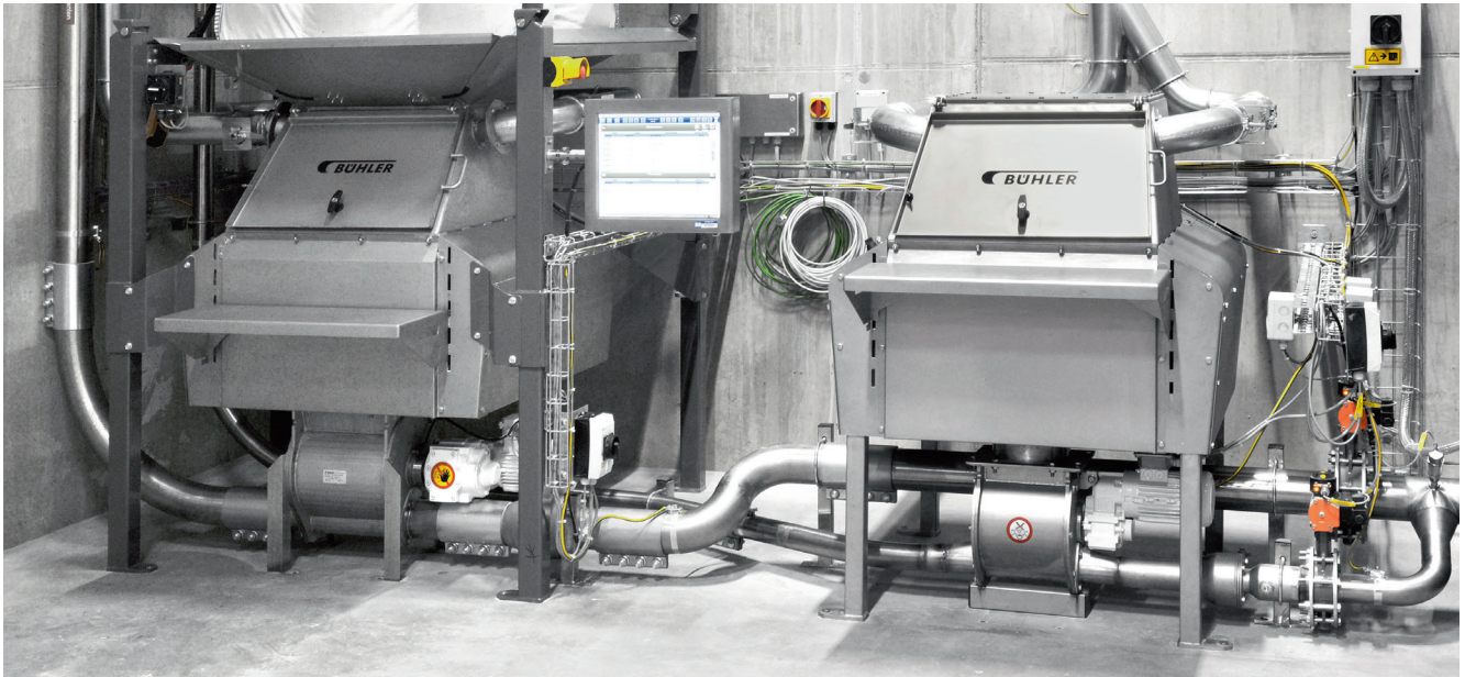
Product feed into the pneumatic conveying line: a blow-through airlock MPSS is used as feeding element below the discharge station MKSB.
