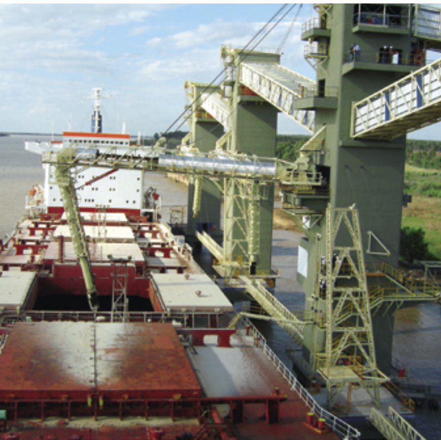
Bunge S.A., Ramallo – Buenos Aires, Argentina. 2 loading lines with a throughput of 1600 t/h, 4 loading towers.
