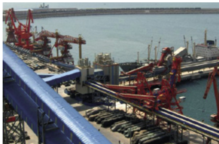
Dalian Beiliang Grain Terminal, China. Efficient and modern Grain Terminal with 2 Buhler ship loaders Portaloader ( 2 \times 1000 t/h) and 2 Buhler ship unloaders Portalink ( 2 \times 1000 t/h) as well as with belt conveyors.
