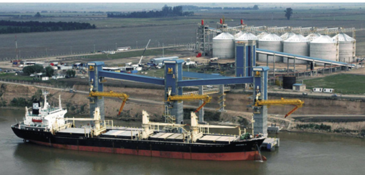
Noble Argentina S.A. – Río Paraná, Argentina. 3 loading towers, 2 loading lines with throughputs of 1600 t/h of soybeans each.
